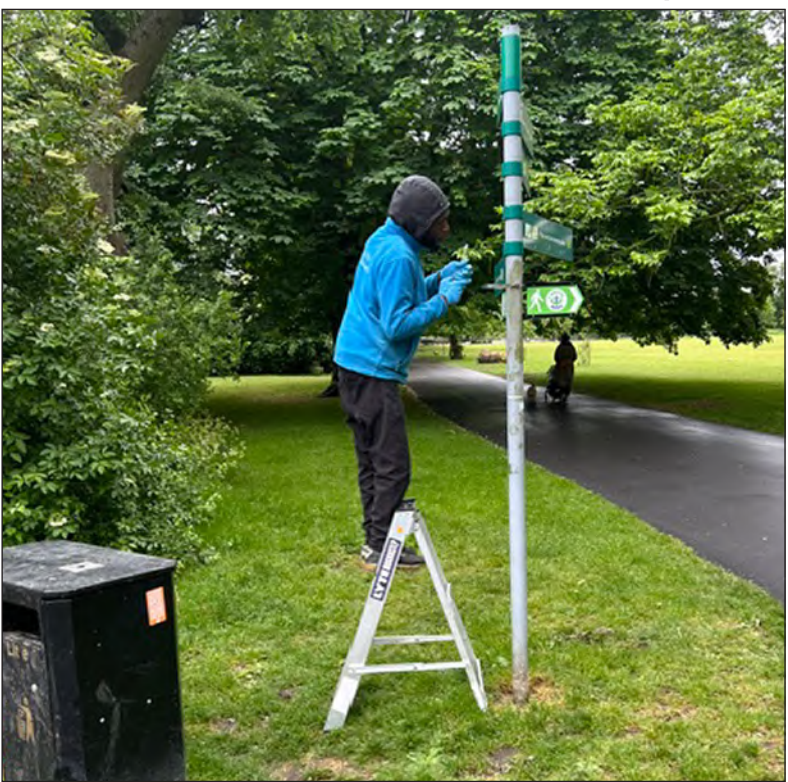
Installing new Capital Ring signing in Clissold Park, Stoke Newington.
