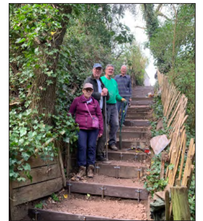
Work on the steps is completed. Photo: Martin Childs
